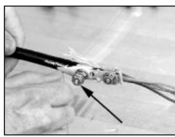
3.13 Finished Scotchlok<sup>TM</sup> 4460-D\FO Shield Bond Connector Assembly on loose tube cable.
