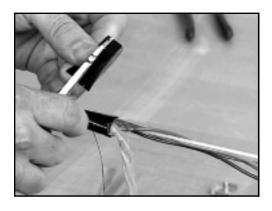
3.4 Insert the fiber protector between the metal cable shield and core wrap to a distance near or equal to its own length.
