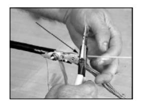
3.8 Dual metallic strength members should be routed through the slots in the extension bracket and folded over.
