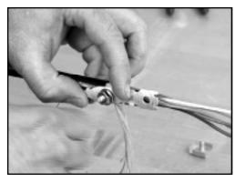
3.7 Single strength members and dual dielectric strength members should be trimmed slightly shorter than the top of the extension bracket.
