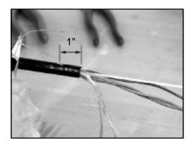
3.3 Cut or trim the plastic fiber protector along it's length to suit the cable jacket size and trim a point on one end.
