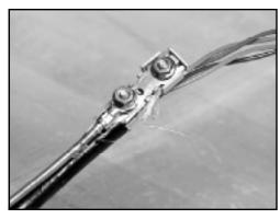
3.14 Finished Scotchlok<sup>TM</sup> 4460-D\FO Shield Bond Connector Assembly on single tube cable.
