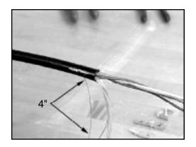
3.2 Using the ripcords for the poly sheath, proceed to slit one inch (2.5 cm) of the jacket open on both sides of the cable. This will allow enough room around the central buffer tube or single buffers for the Scotchlok <sup>™</sup> 4460-D\FO Shield Bond Connector Assembly to be installed.
