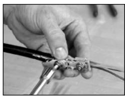
3.12 Add the third securing nut to the connector bottom stud only for adding any ground wires or straps.
